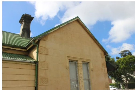
Figure : Rendered quoins on the south west elevation of the building
