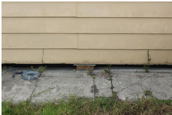
Figure 26: West elevation of enclosed verandah clad in Hardi plank boards with brick footings.
