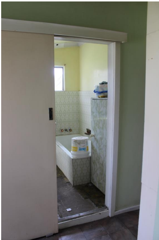
Figure 43: Contemporary bathroom fitout at the rear of the house
