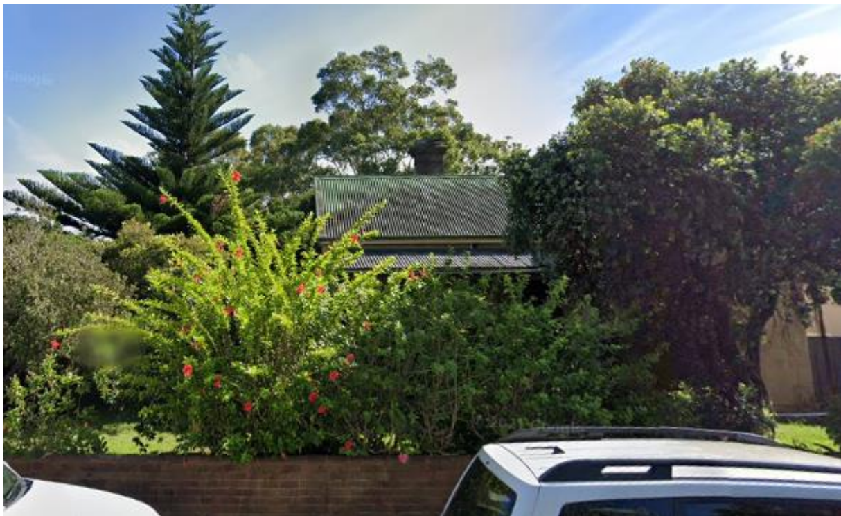
Figure 45: 14 Sunderland Street viewed from the south prior to removal of vegetation. Source: Google Street view 2021
