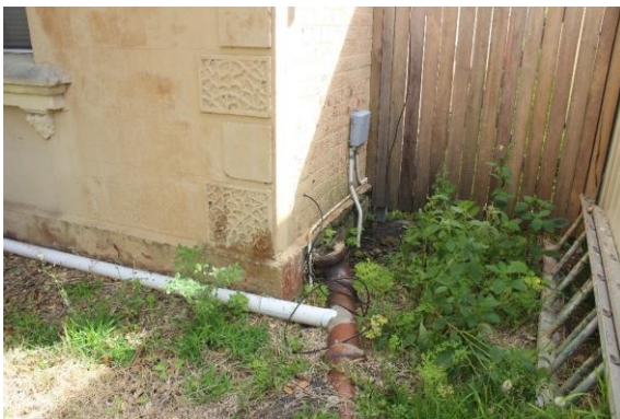
Figure 22: Rendered quoins on the south east corner of the building
