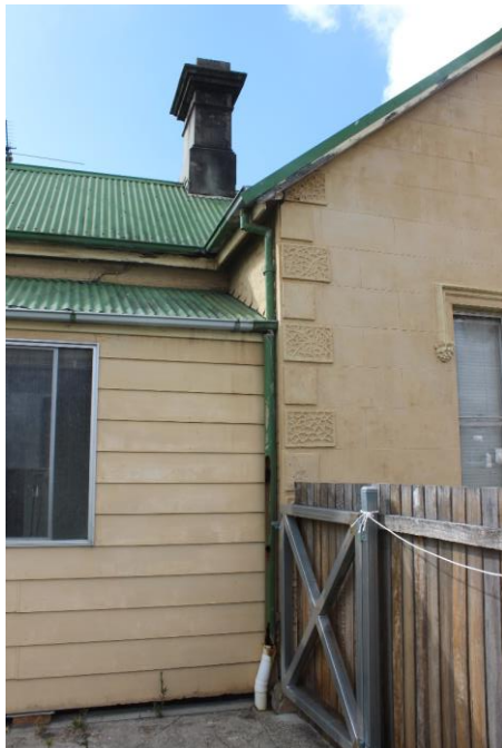
Figure 27: West elevation of enclosed veranda clad in Hardi plank boards with timber fence and gate.
