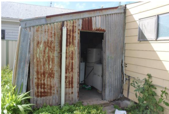
Figure 25: Rear skillion laundry addition clad in corrugated galvanised steel
