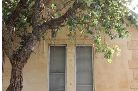
Figure 21: Label mould and cast decorative mouldings on the Sunderland Street façade.
