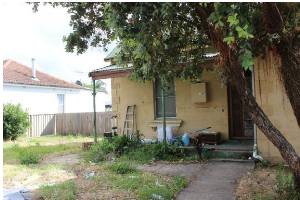
Figure 19: View north to front porch
