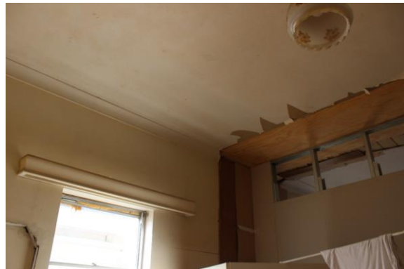
Figure 38: Partial removal of wall between the rooms.
