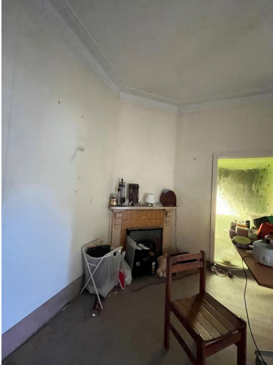
Figure 41: Remaining fireplace in the western back room.
